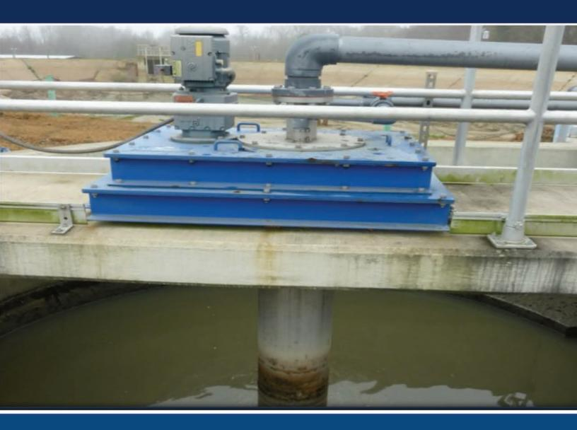
Providing Efficient and Low Maintenance 95% Grit Removal Since 1977
